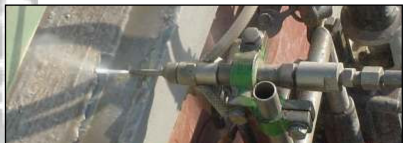
Photo above: Detail of cutting a tank roof off the tank.
