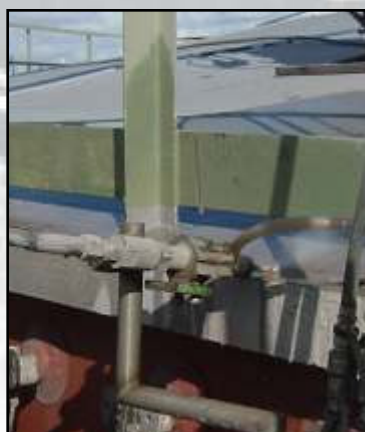
Photo above: Detail of cutting a tank roof off the tank.
